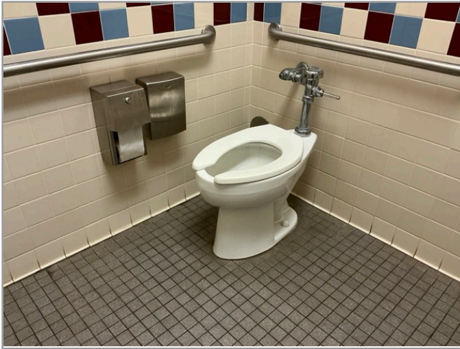
TOILET STALL OVERVIEW
