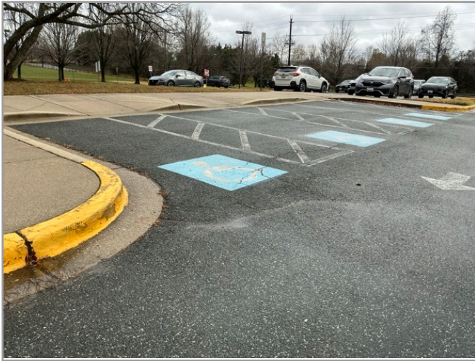
OVERVIEW OF ACCESSIBLE PARKING AREA
